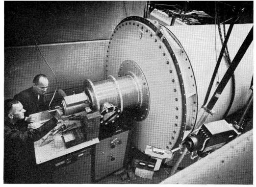
HERMES I, a one-tenth scale model of HERMES II, was built to help solve the complex problems involved in creating the world's largest flash x-ray generator. The model is now a useful device in Sandia's radiation effects program. Jim Maxim, left, and Ralph Schellenbaum operate the machine.
